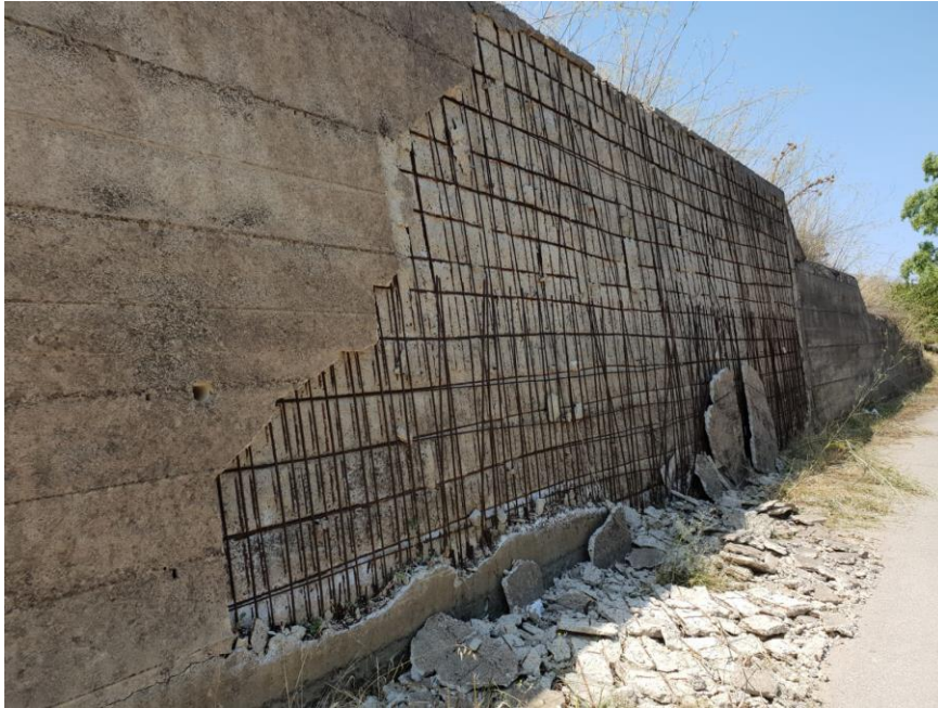
[R. Maddalena, 2018 – Retaining wall, SS560, ITALY]
